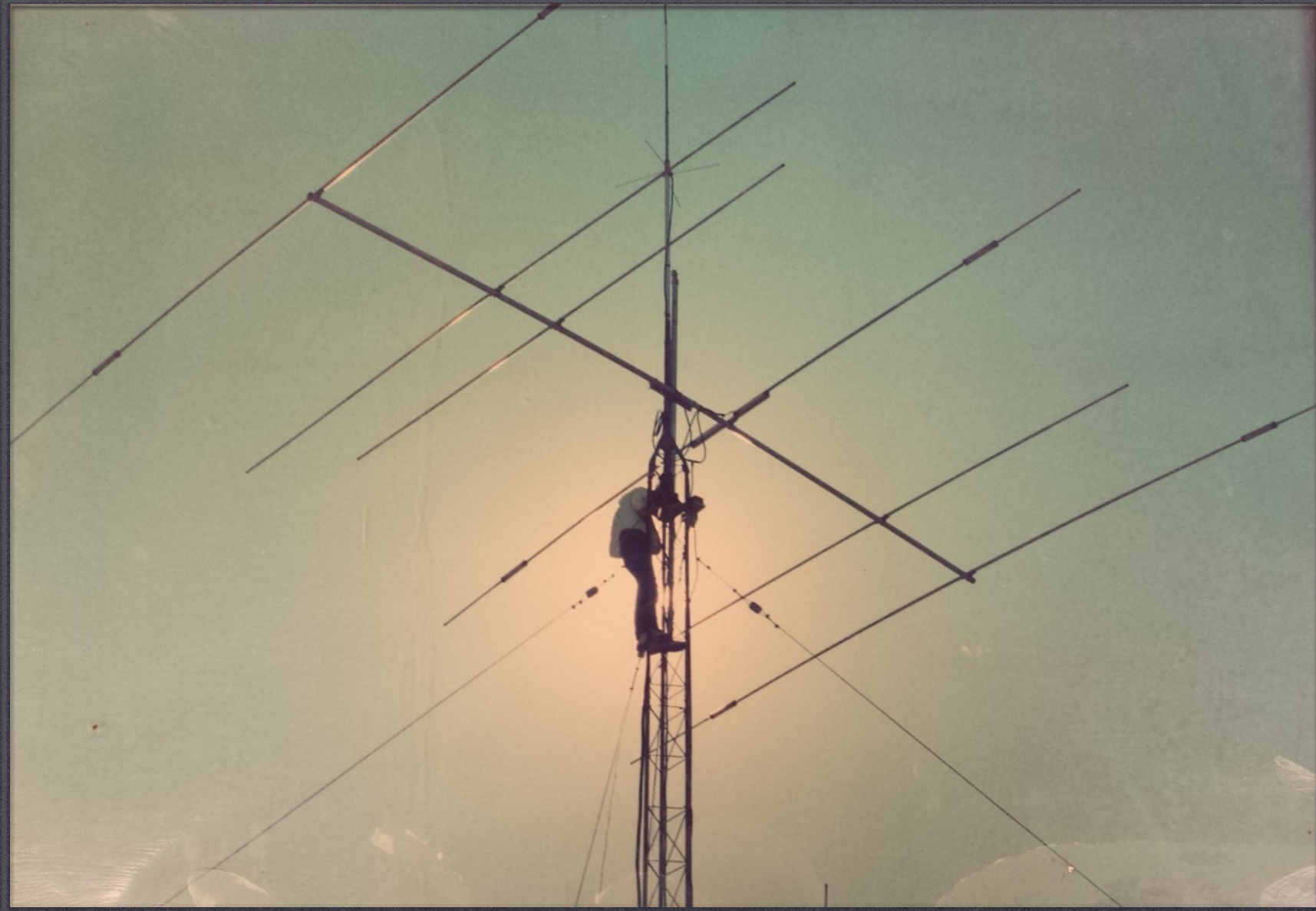
Main Tower - 60 ft. Rohn 25G South Campus Dining Facility
